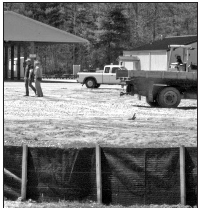
Construction of expanded facilities at the Union County Farmers Market are on schedule. Photo/Todd Forrest
